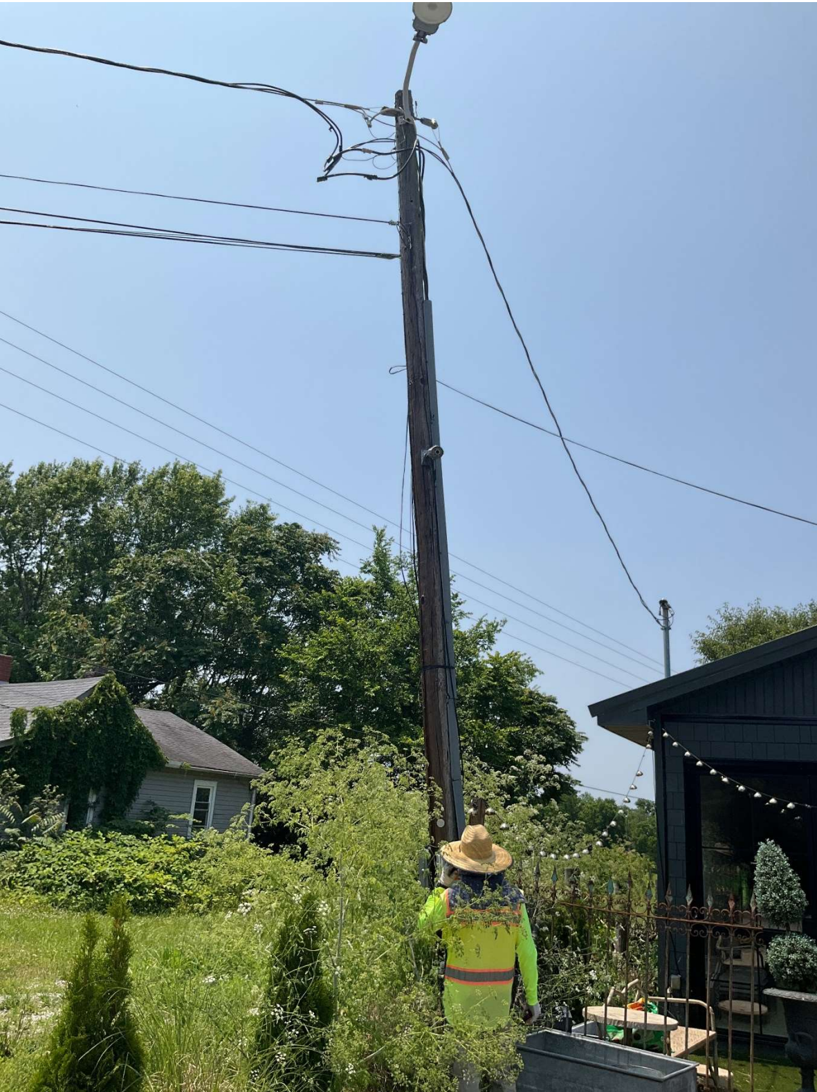
Communications attachments are above the top of the electric service riser in the power space.
